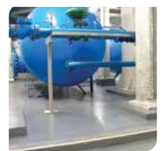
Plant Rooms and Maintenance
