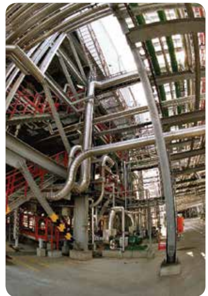
Metal structure coatings
